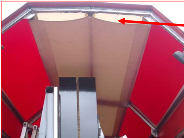
Cotton tarpaulin in order to avoid from condensation
